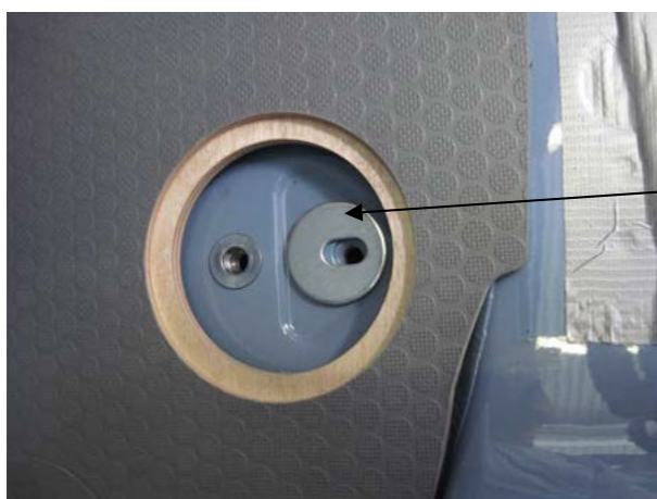
Drill hole using a step drill; make it even using a large washer (not included in delivery)
