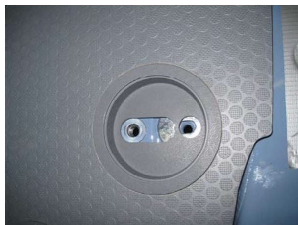
Drill hole using a step drill; make it even using a large washer (not included in delivery)
